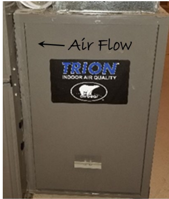
Figure 21-1. Furnace Air Flow Direction.
