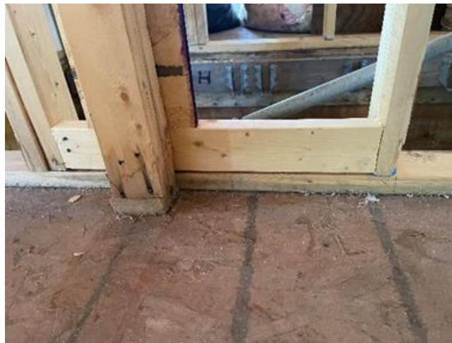
Figure 10-9. Closet Wall Blocking.
