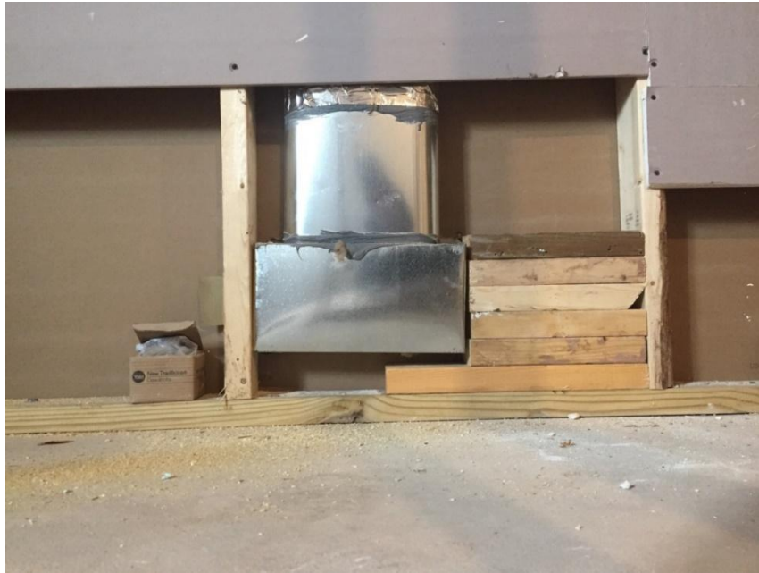
Figure 10-10. Cold Air Return Blocking.
