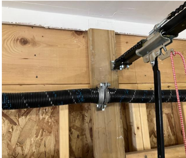
Figure 10-11. OHD Center Blocking.
