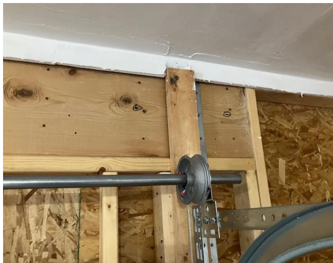
Figure 10-12. OHD Edge Blocking
