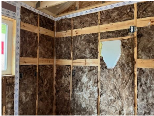
Figure 10-4. Kitchen Cabinet Blocking
