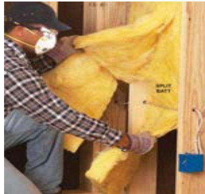
Figure 12-7. Insulating Around Electrical Wires.
