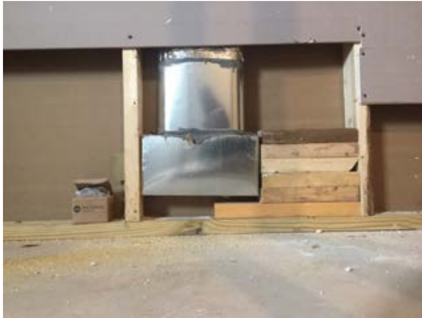
Figure 10-10. Cold Air Return Blocking.
