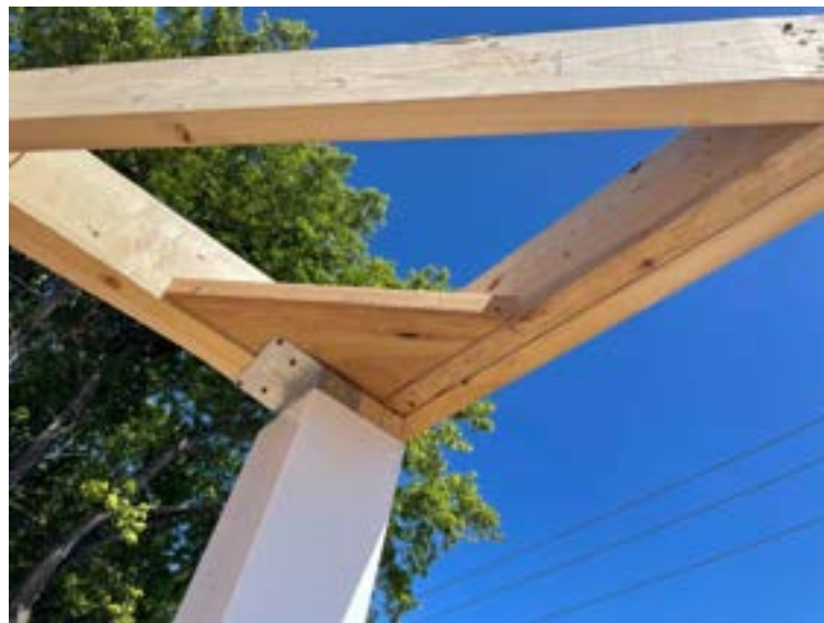
Figure 6-3. Porch Post Trim Ring Blocking.
