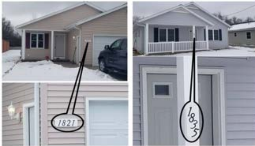
Figure 20-3. House Numbers Installed on a Board.
