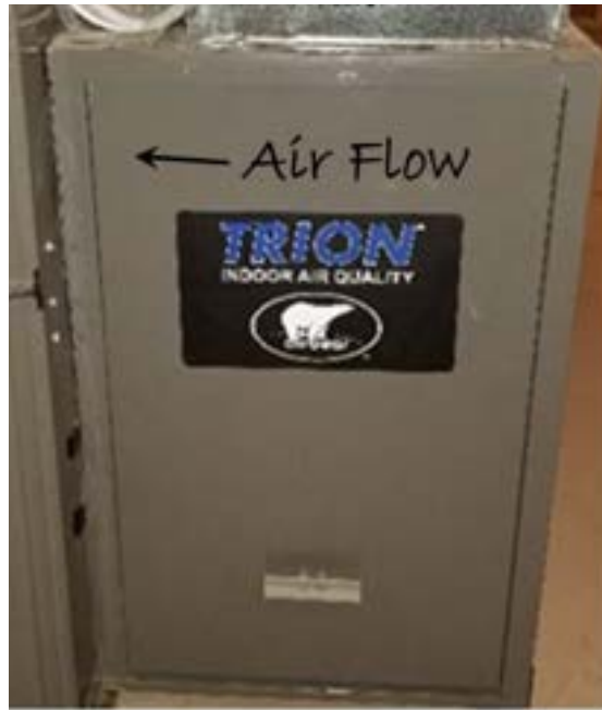
Figure 21-1. Furnace Air Flow Direction.
