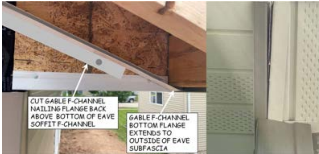
Figure 11-6. F-Channel at Gable Corner.
