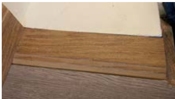
Figure 19-3. Stairway Trim Finish With Ledge.
