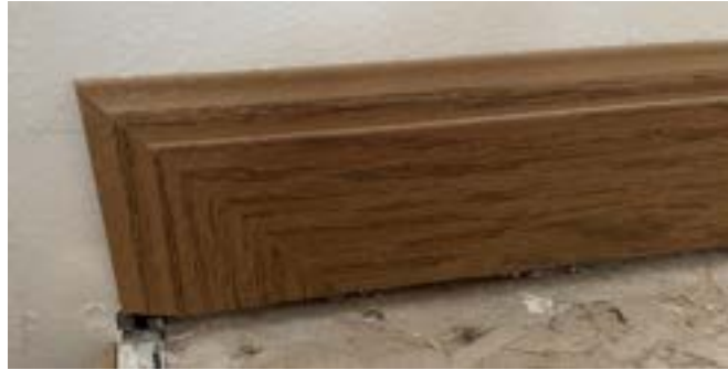
Figure 19-1. Trim End Finish in Closet Platform.
