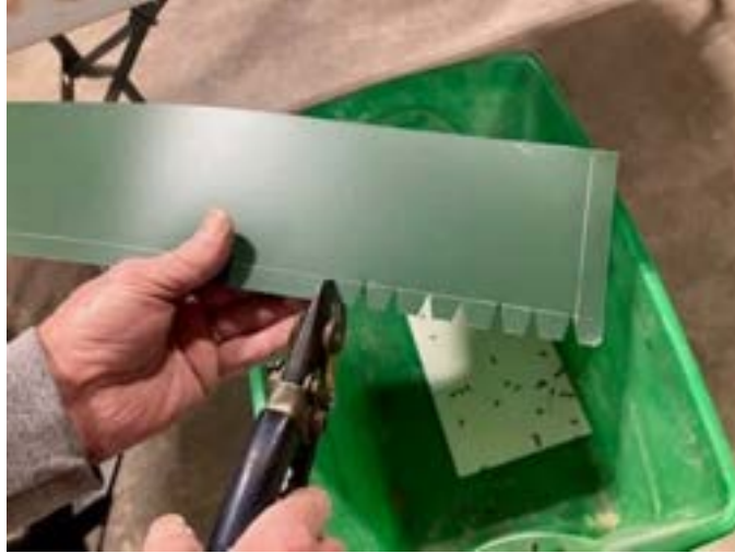
Figure C-14. Plenum Exhaust Pipe.
