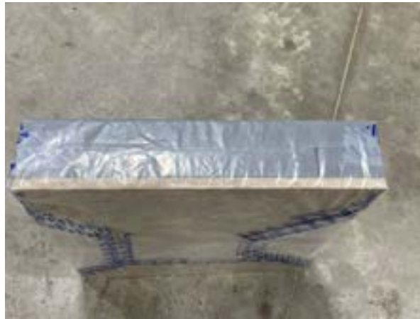
Figure 7-6. House Scuttle Cover Assembly.
