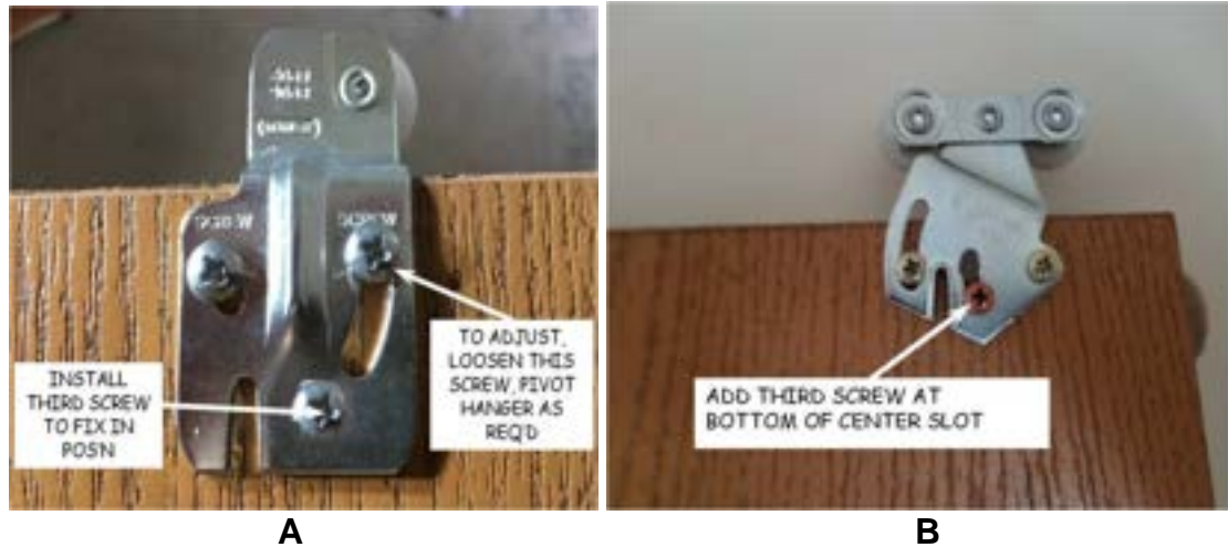
Figure 18-4. Closet Door Hanger with 3 rd Screw Installed.
