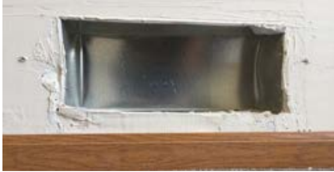
Figure 19-11. Sealing Plaster Gaps Around Cold Air Returns
