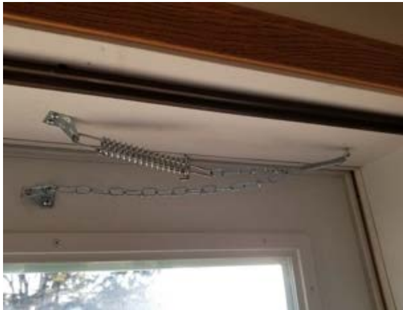
Figure 20-1. Storm Door Wind Chain.
