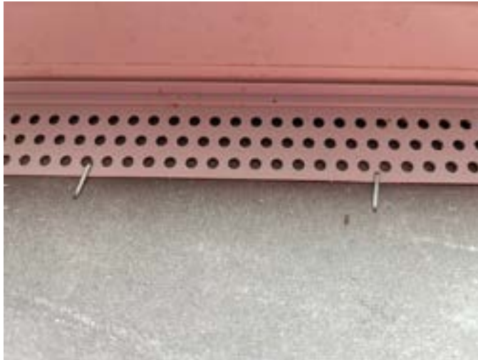
Figure 14-9. Final Staple Securement of Edging Strips.
