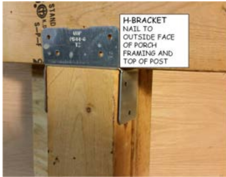
Figure 6-2. Porch Post H-Bracket.
