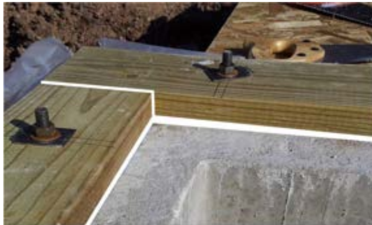
Figure 1-3. Sill Plate Installation.
