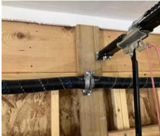
Figure 10-11. OHD Center Blocking.
