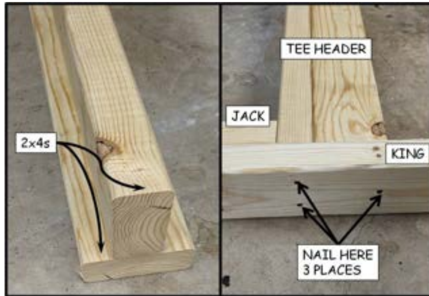
Figure 4-3. T-Header Assembly.
