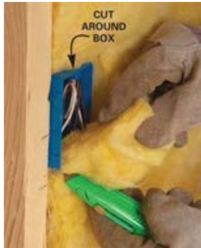
Figure 12-8. Insulating Around Electrical Box.
