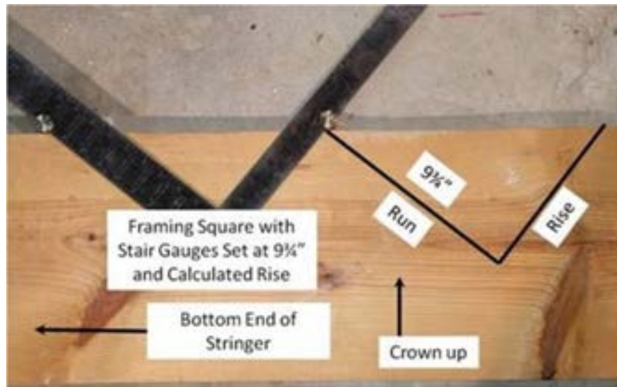
Figure 4-6. Stair Stringer Layout.
