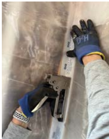
Figure 12-11. Pushing Poly Into The Corner While Stapling.
