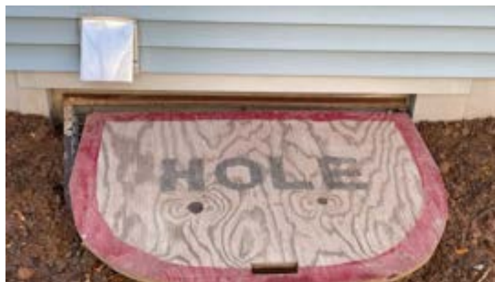
Figure 11-3. Skirting Around Egress Window.
