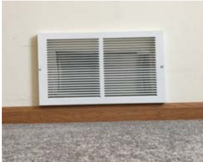
Figure 19-12. Positioning Cold Air Return Vent Covers.
