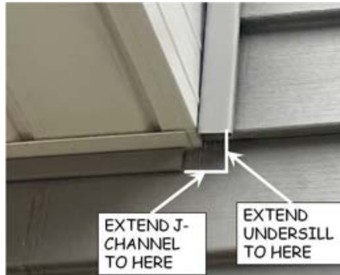
Figure 11-10. Undersill/J-Channel Corner.
