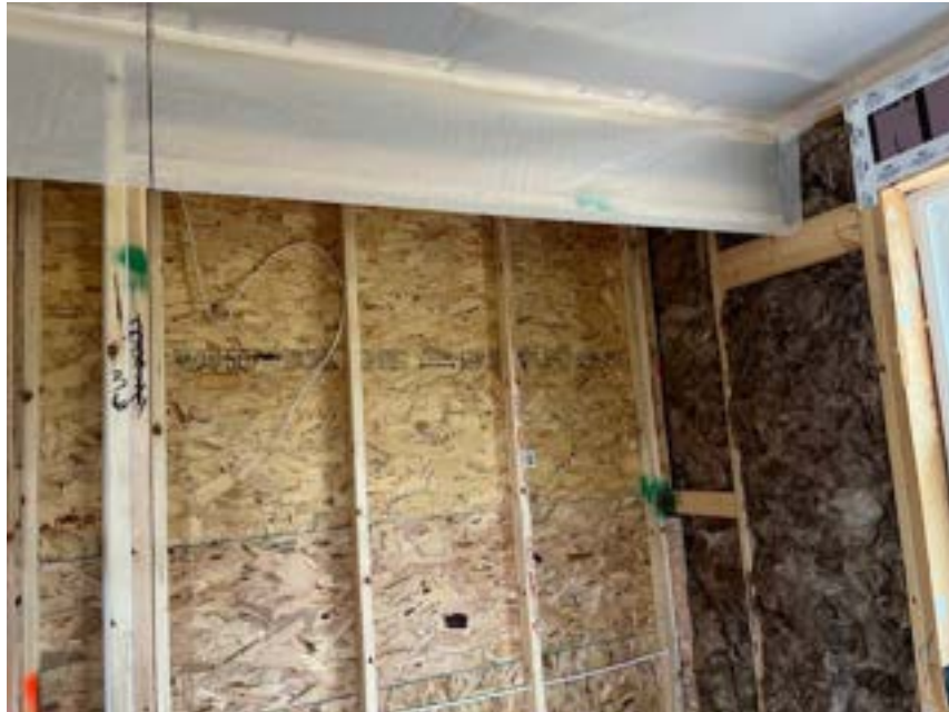
Figure 12-9. Extend Ceiling Poly to Cover Flush Closet Header.
