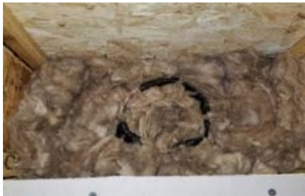
Figure 12-2. Insulation Filled Around Future Fan Vent Duct.
