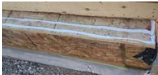
Figure 5-3. Air Sealing Caulk.
