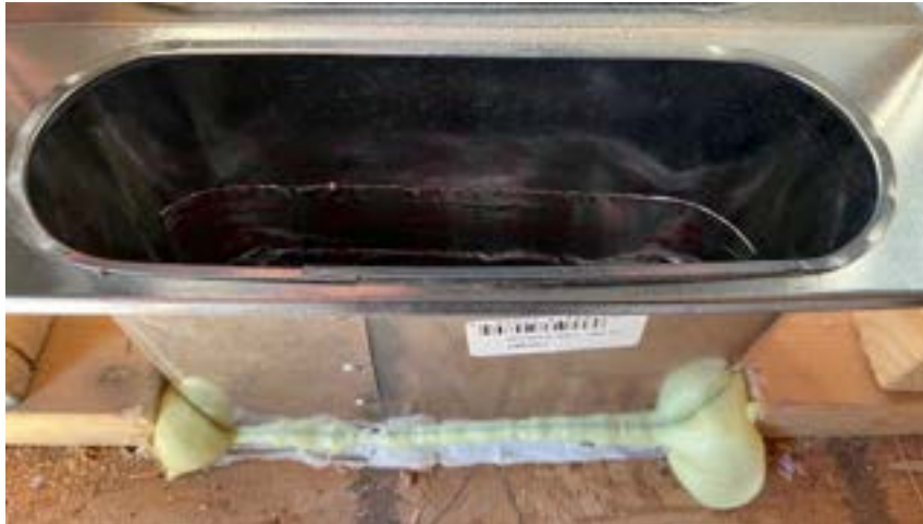
Figure 12-5. Sealing Cold Air Return Joints
