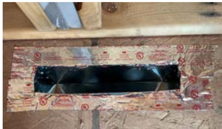
Figure 12-4. Sealing In-Floor Heating Duct.
