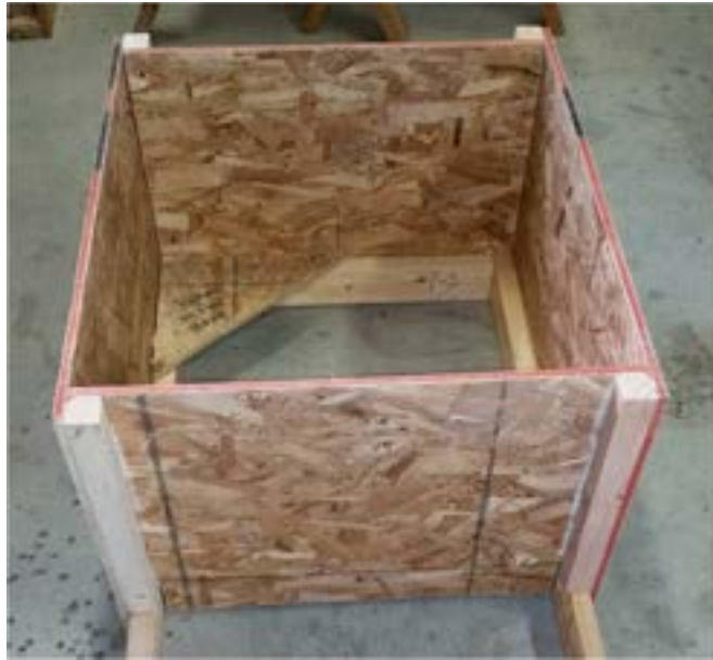
Figure 7-3. House Scuttle Box.
