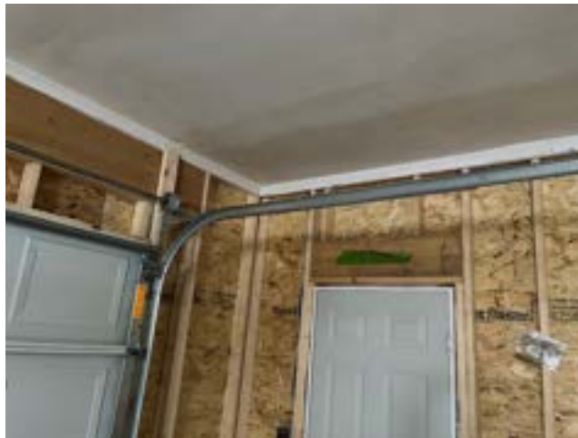
Figure 13-6. Covering Garage Exterior Wall Plates.
