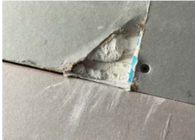
Figure 13-2. Broken Corner.
