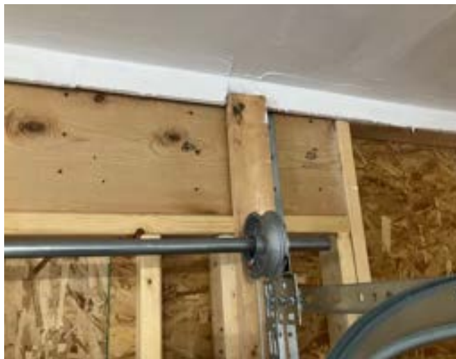
Figure 10-12. OHD Edge Blocking
