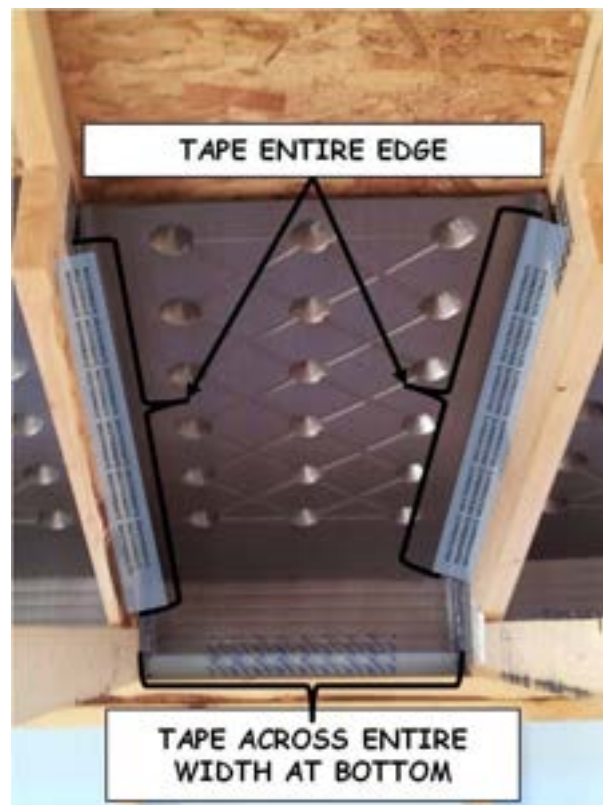
Figure 10-3. Proper Vent Installation.
