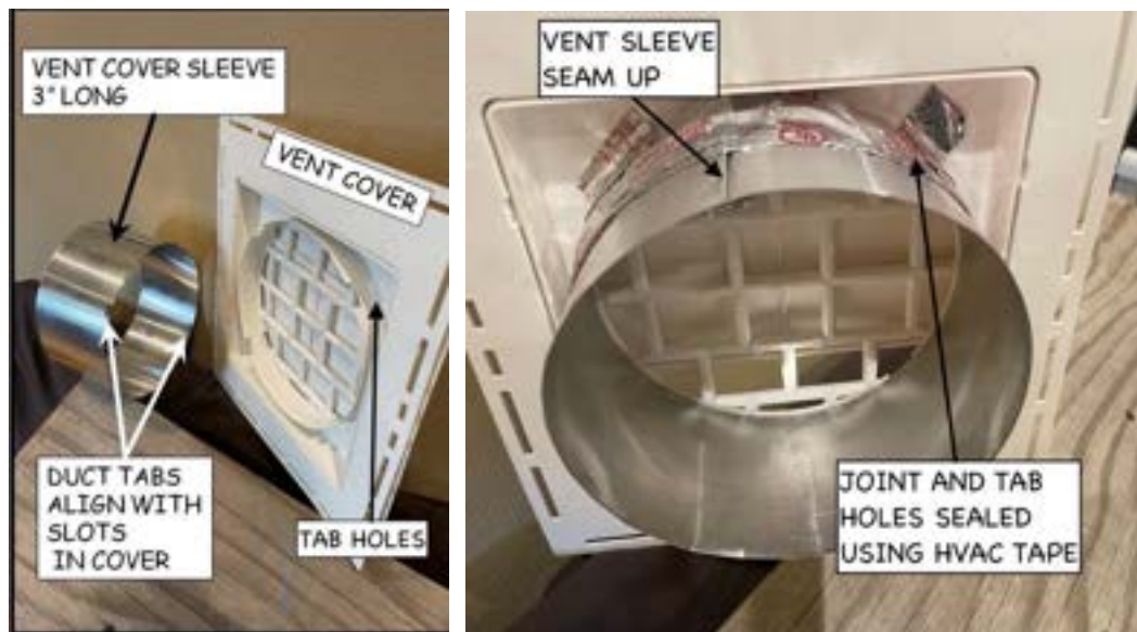
Figure 10-2 – Range Vent Cover Sleeve Assembly
