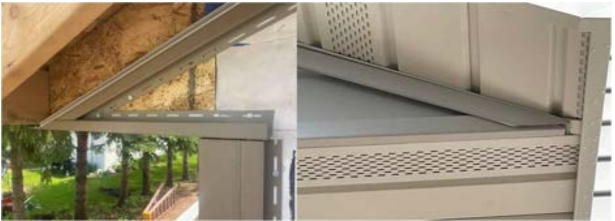
Figure 11-8. J-Channel at Gable Corner.
