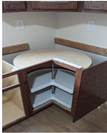
Figure 17-3. Showing Countertop 2x4 Corner Supports.
