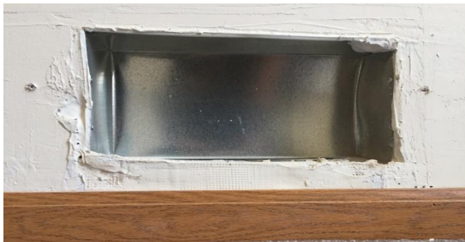
Figure 19-7. Sealing Plaster Gaps Around Cold Air Returns
