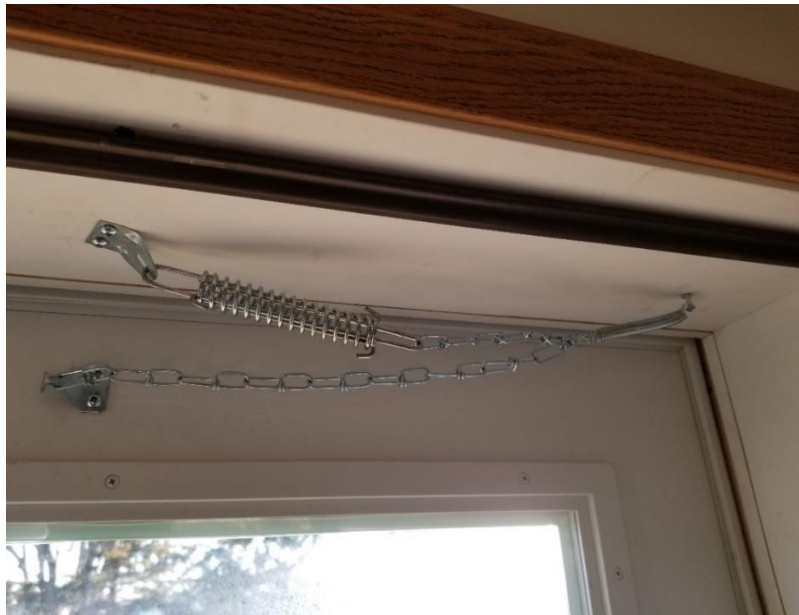
Figure 20-1. Storm Door Wind Chain.
