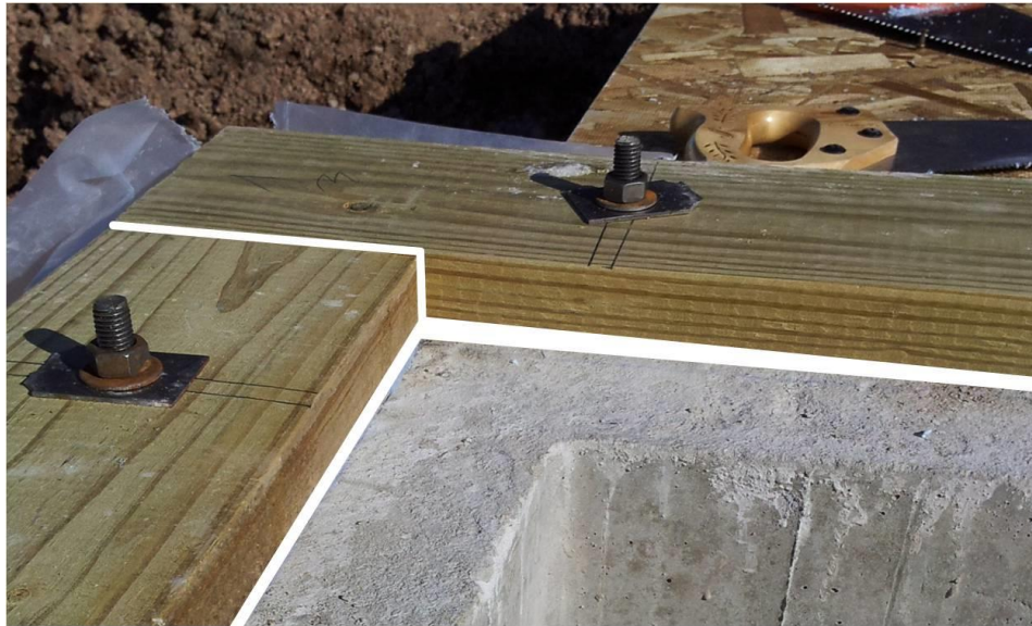
Figure 1-3. Sill Plate Installation.
