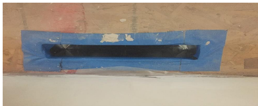
Figure 12-4. Sealing In-Floor Heating Duct.
