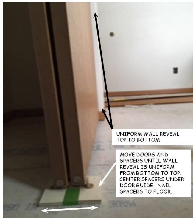
Figure 18-4. Shim Adjustment for Uniform Door Reveal.
