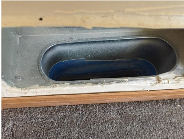
Figure 12-5. Sealing Cold Air Return Joints
