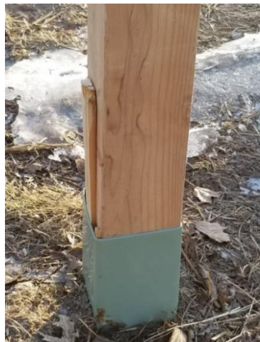
Figure 20-3. Installation of Mailbox Post.
