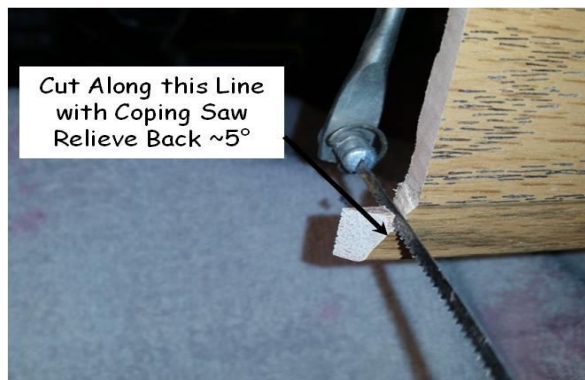
Figure 19-4. Coping Saw Cut.
