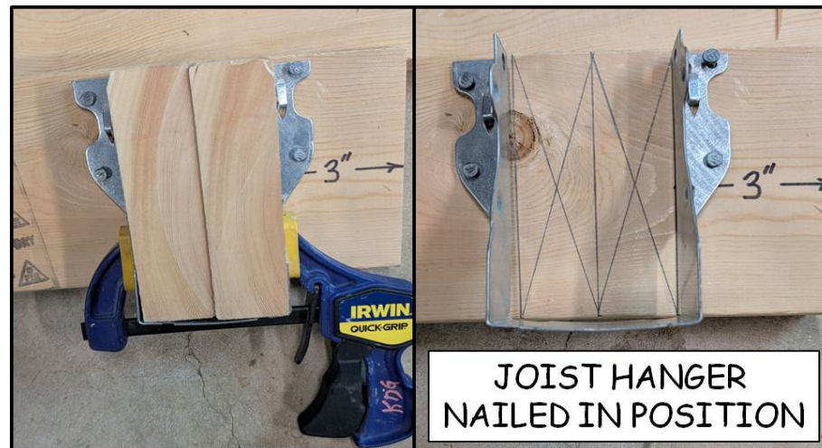
Figure 6-2. Porch Side Frame Joist Hanger.
