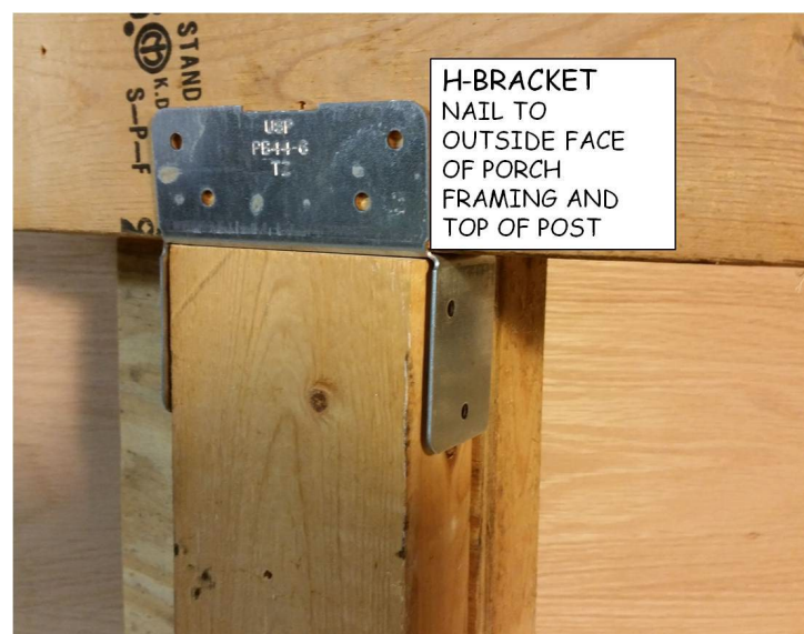
Figure 6-5. Porch Post H-Bracket.
