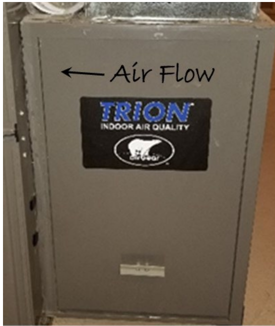
Figure 21-1. Furnace Air Flow Direction.
