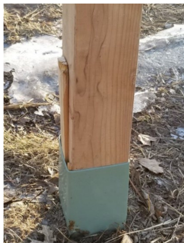
Figure 20-4. Installation of Mailbox Post.
