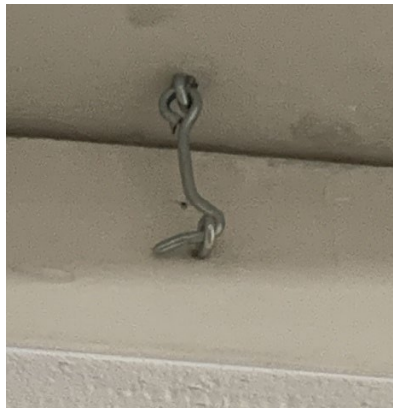
Figure 19-13. Garage Scuttle Cover Hook and Eye Assembly.
