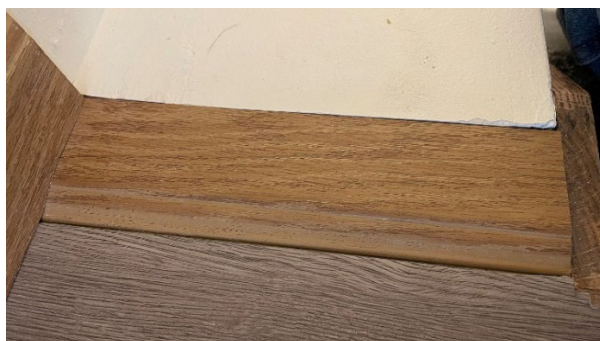
Figure 19-3. Stairway Trim Finish With Ledge.
