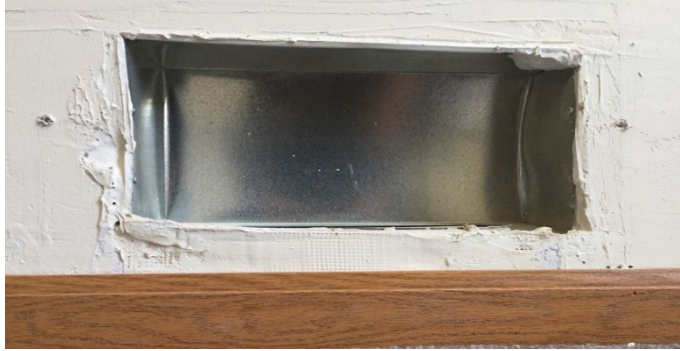
Figure 19-11. Sealing Plaster Gaps Around Cold Air Returns
