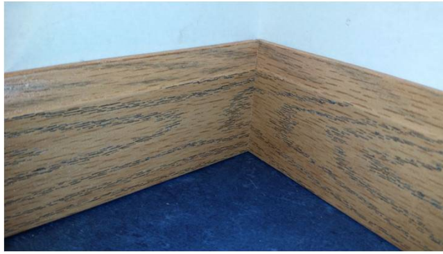
Figure 19-9. Finished Coped Joint.
