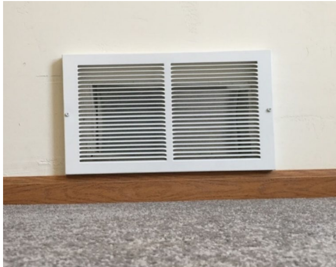
Figure 19-12. Positioning Cold Air Return Vent Covers.
