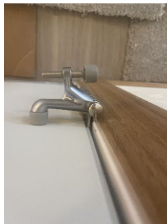
Figure 18-1. Correct Bumper Orientation.
