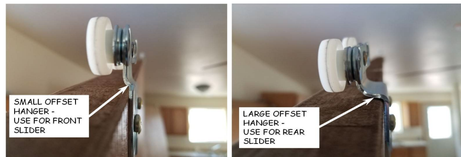
Figure 18-2. Sliding Door Hangers.
