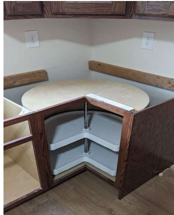
Figure 17-3. Showing Countertop 2x4 Corner Supports.
