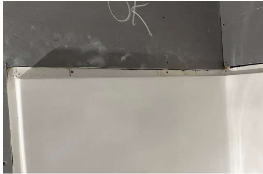
Figure 14-13. Sheetrocking Around Tub/Shower Nailing Flange.
