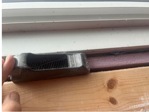
Figure 14-1. Trimming Foamboard Around Basement Window.
