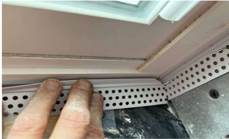
Figure 14-11. 45° Clipped Corners and Inside Row Hole Stapling.
