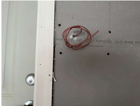
Figure 14-9. Pulling Wires Through Sheetrock.
