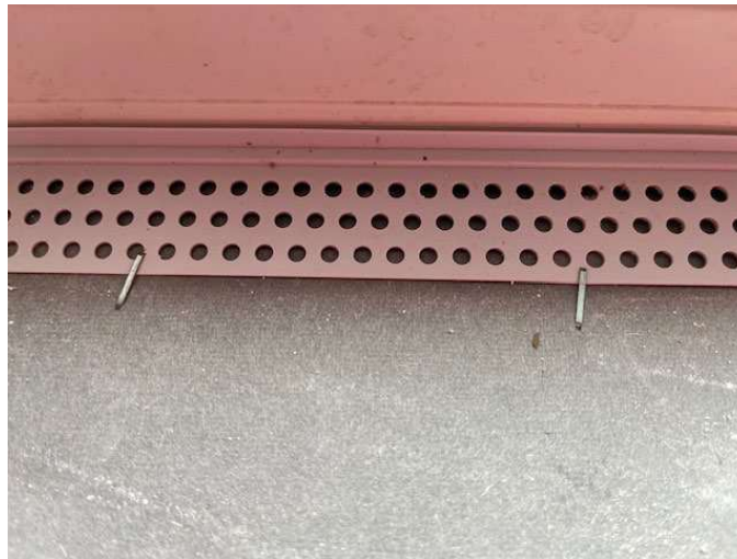
Figure 14-12. Final Staple Securement of Edging Strips.
