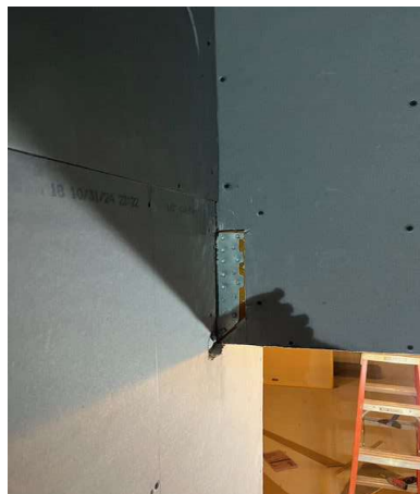
Figure 14-10. Trimming Around Joist Hangers.
