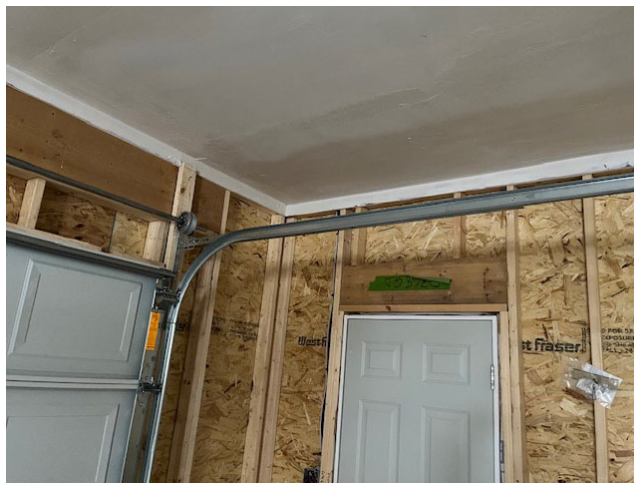
Figure 13-7. Covering Garage Exterior Wall Plates.
