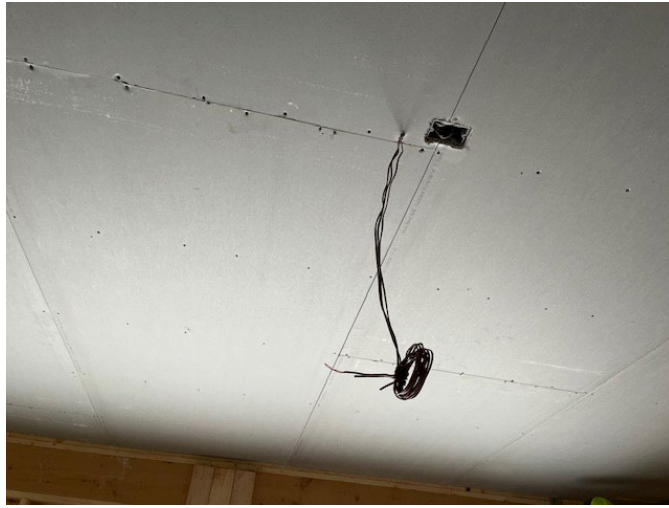
Figure 13-6. Exposing Garage Door Opener Wire.
