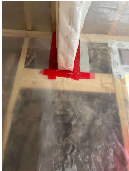
Figure 12-12. Air Sealing Around a Flush Closet Header.
