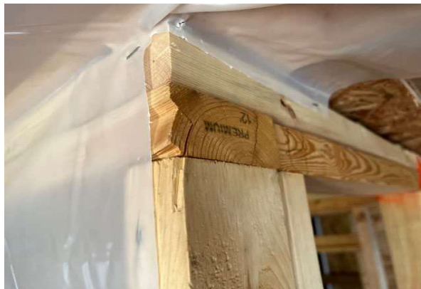
Figure 12-10. Extending Poly Around a Corner.
