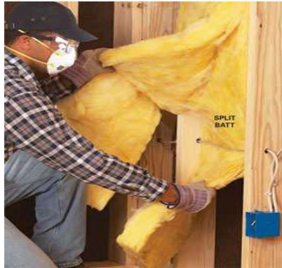
Figure 12-7. Insulating Around Electrical Wires.
