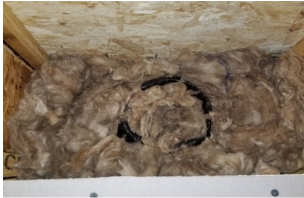
Figure 12-2. Insulation Filled Around Future Fan Vent Duct.
