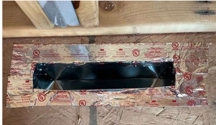
Figure 12-4. Sealing In-Floor Heating Duct.
