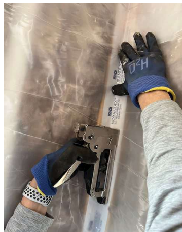
Figure 12-11. Pushing Poly Into The Corner While Stapling.
