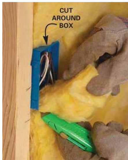
Figure 12-8. Insulating Around Electrical Box.
