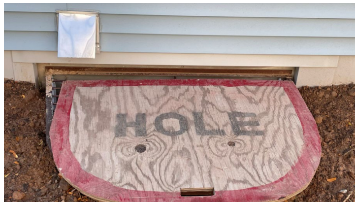
Figure 11-3. Skirting Around Egress Window.
