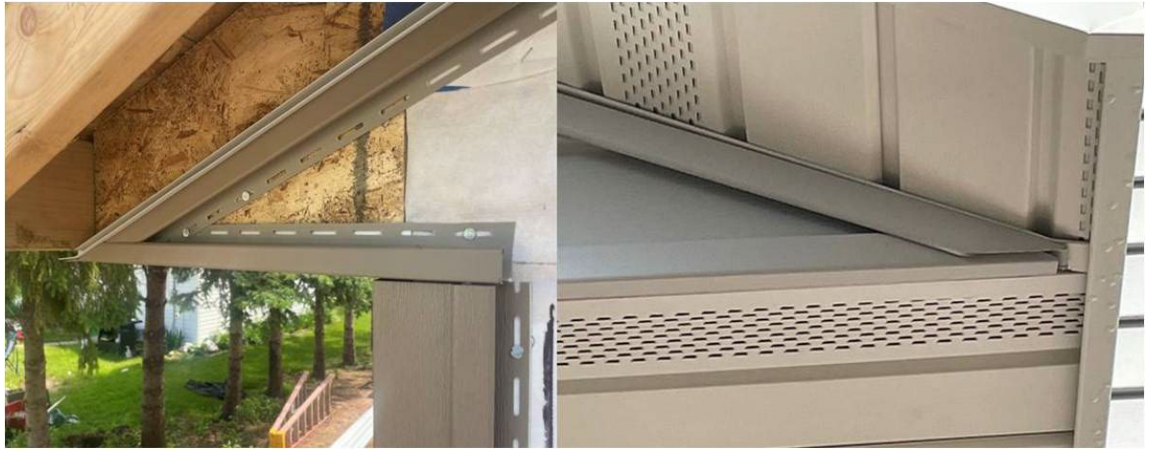
Figure 11-8. J-Channel at Gable Corner.
