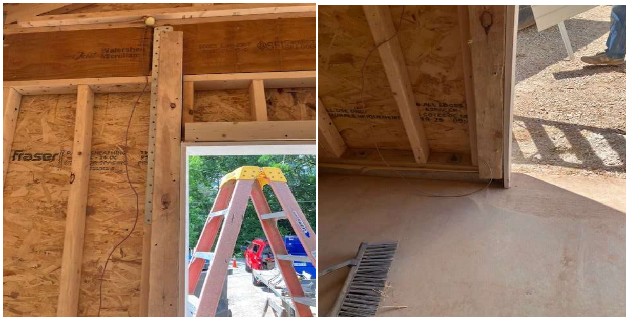
Figure 10-12. OHD Edge Blocking.
