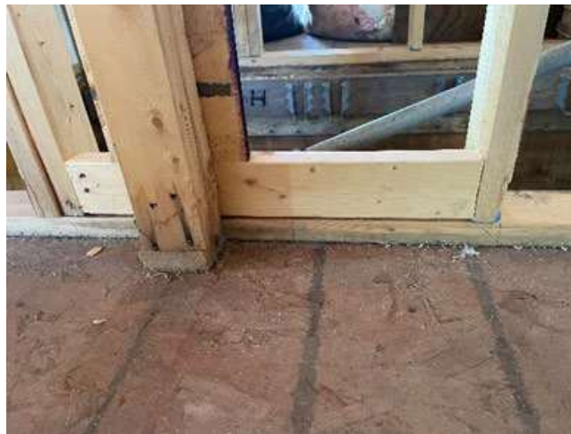
Figure 10-9. Closet Wall Blocking.
