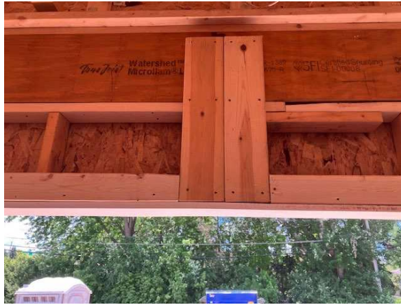
Figure 10-11. OHD Center Blocking.
