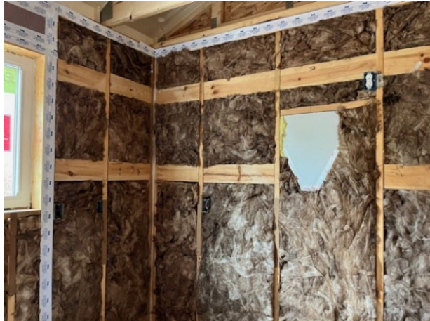
Figure 10-4. Kitchen Cabinet Blocking
