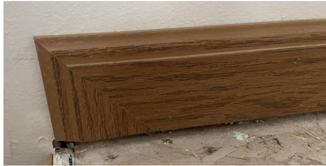
Figure 19-1. Trim End Finish in Closet Platform.
