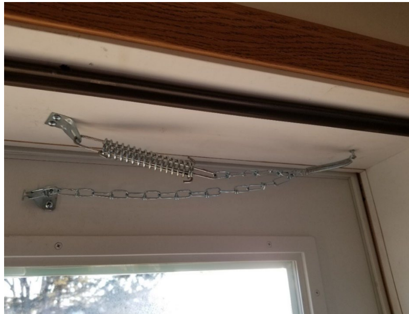
Figure 20-1. Storm Door Wind Chain.
