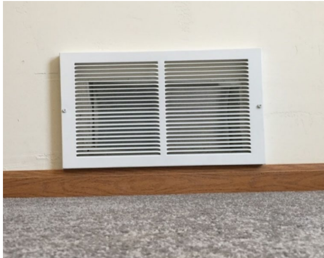
Figure 19-12. Positioning Cold Air Return Vent Covers.
