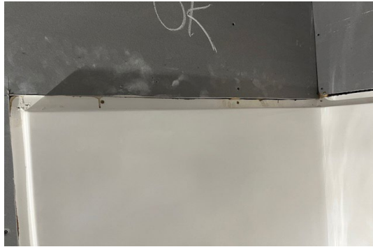
Figure 14-13. Sheetrocking Around Tub/Shower Nailing Flange.
