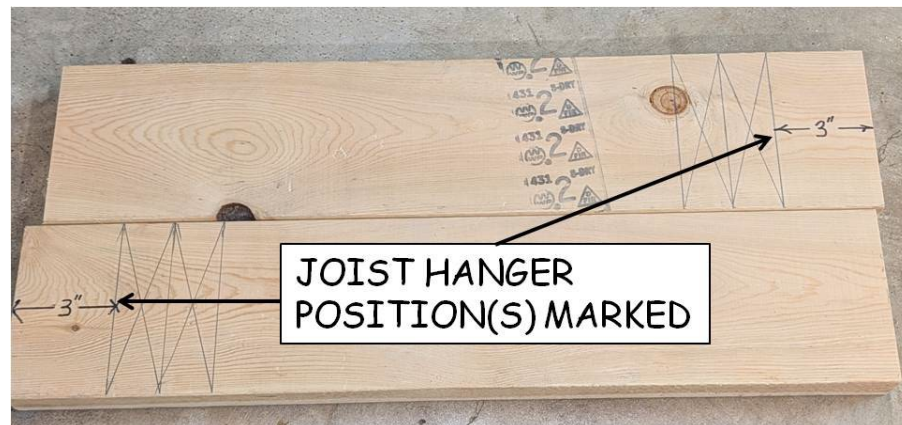
Figure 6-1. Joist Hanger Cleats.
