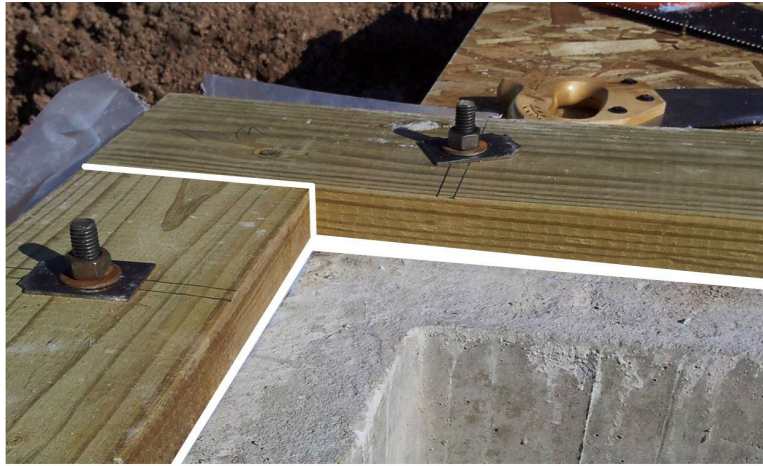
Figure 1-3. Sill Plate Installation.
