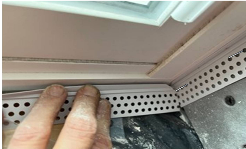
Figure 14-11. 45° Clipped Corners and Inside Row Hole Stapling.
