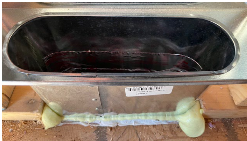
Figure 12-5. Sealing Cold Air Return Joints
