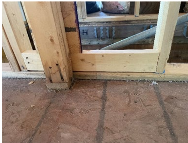
Figure 10-9. Closet Wall Blocking.
