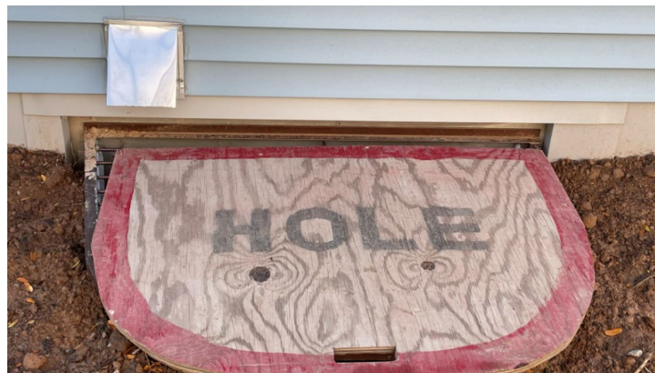
Figure 11-3. Skirting Around Egress Window.
