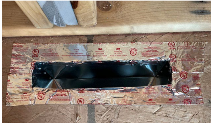
Figure 12-4. Sealing In-Floor Heating Duct.
