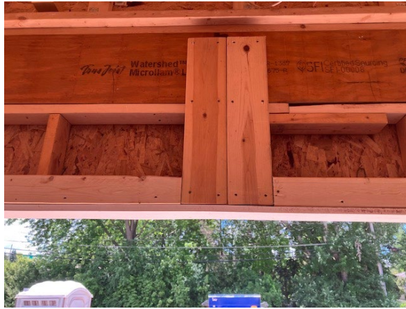
Figure 10-11. OHD Center Blocking.
