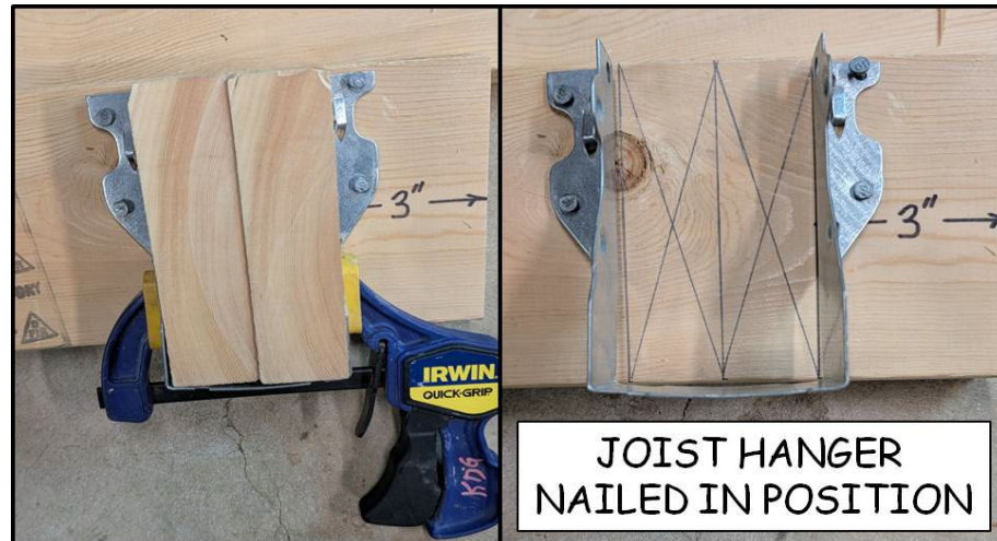
Figure 6-2. Porch Side Frame Joist Hanger.
