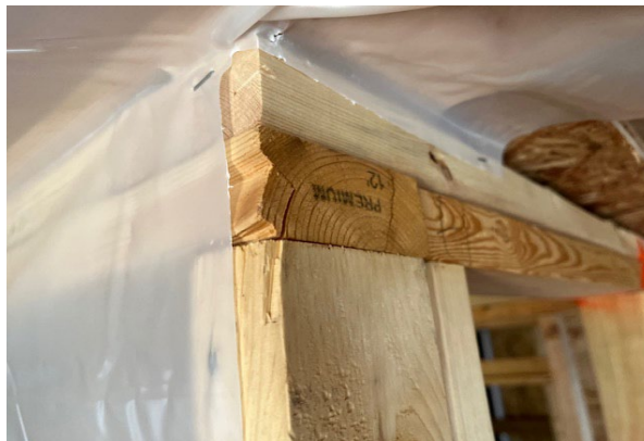
Figure 12-10. Extending Poly Around a Corner.
