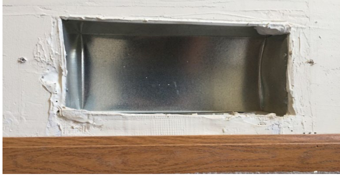
Figure 19-11. Sealing Plaster Gaps Around Cold Air Returns
