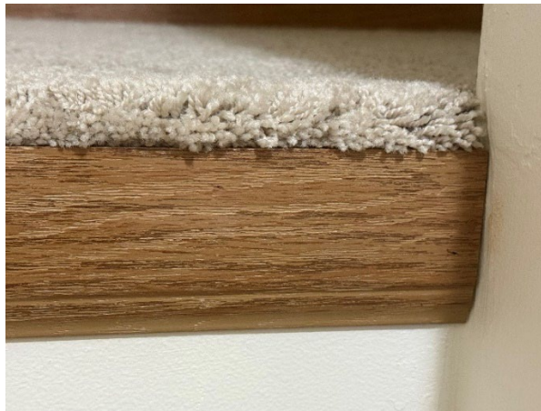
Figure 19-2. Closet Platform Edge Trim After Carpet Installation.
