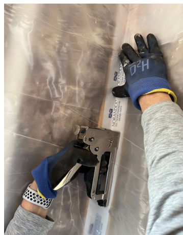
Figure 12-11. Pushing Poly Into The Corner While Stapling.
