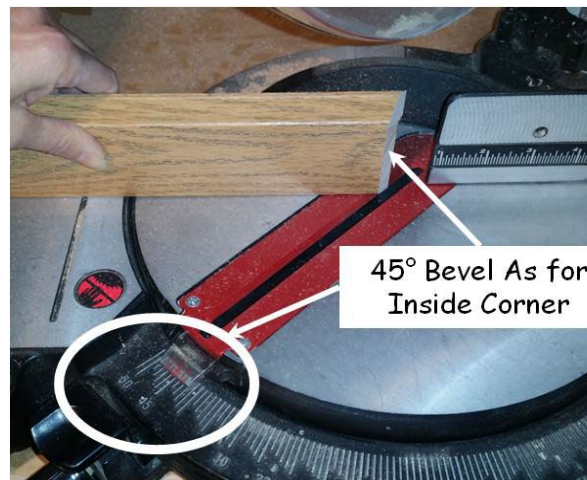
Figure 19-5. Base Trim Bevel Cut.
