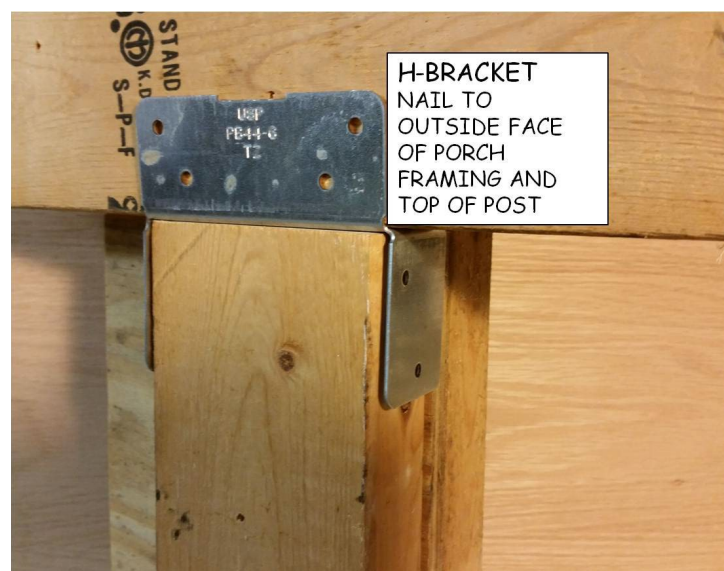
Figure 6-5. Porch Post H-Bracket.
