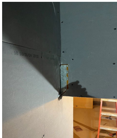
Figure 14-10. Trimming Around Joist Hangers.
