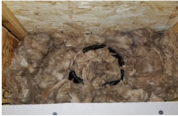
Figure 12-2. Insulation Filled Around Future Fan Vent Duct.
