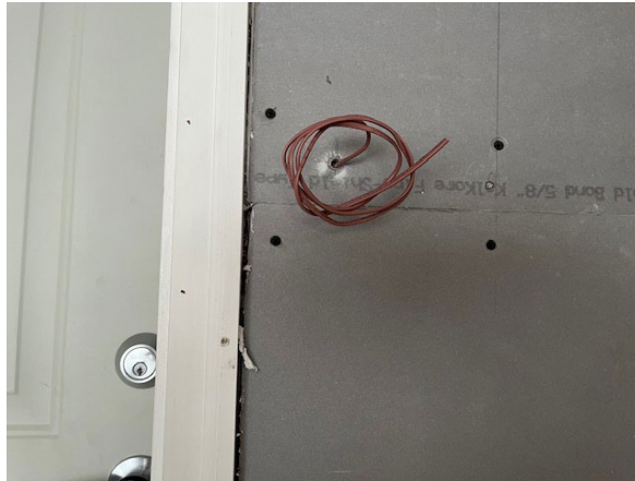
Figure 14-9. Pulling Wires Through Sheetrock.
