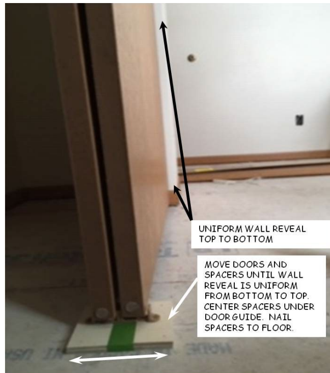
Figure 18-5. Shim Adjustment for Uniform Door Reveal.
