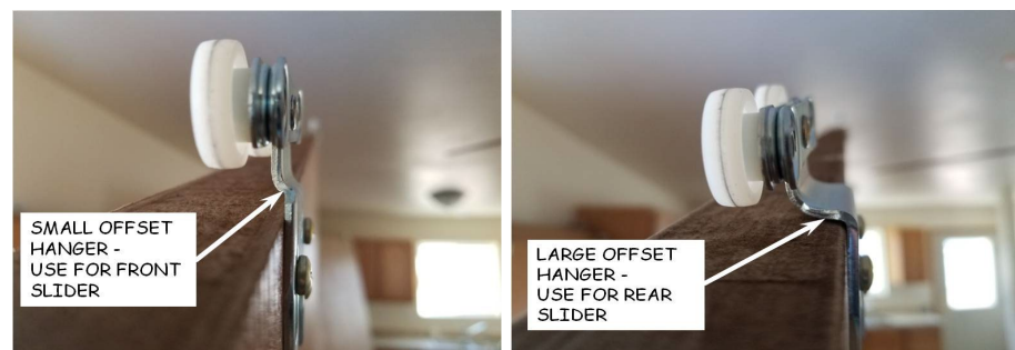
Figure 18-2. Sliding Door Hangers.
