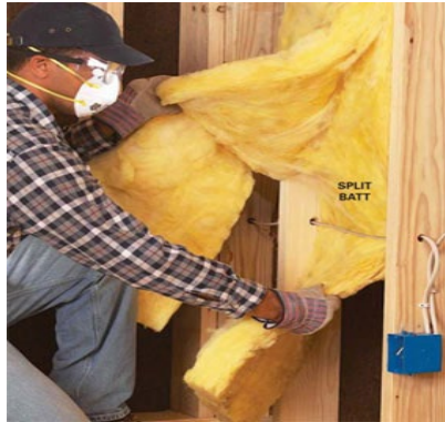
Figure 12-7. Insulating Around Electrical Wires.
