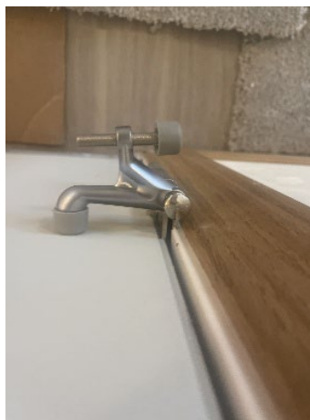
Figure 18-1. Correct Bumper Orientation.
