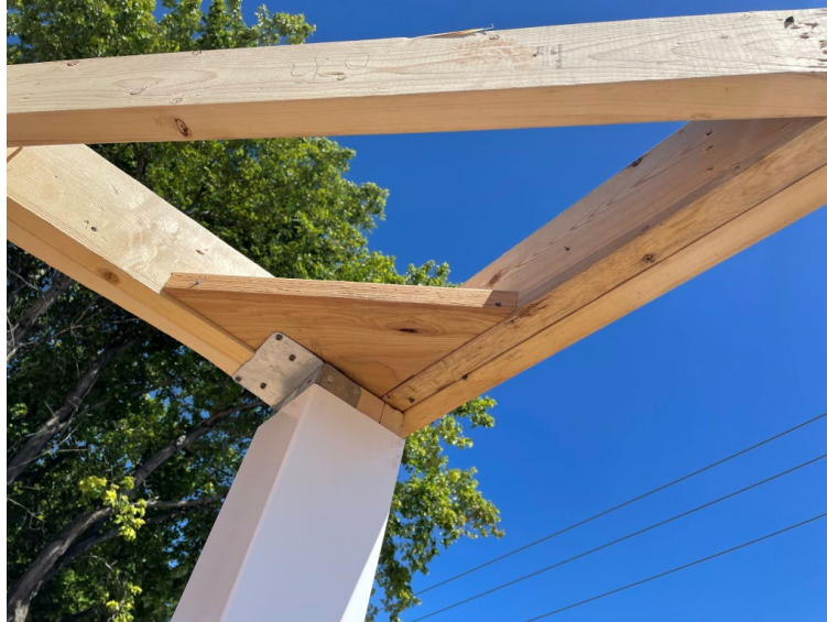
Figure 6-6. Porch Post Trim Ring Blocking.
