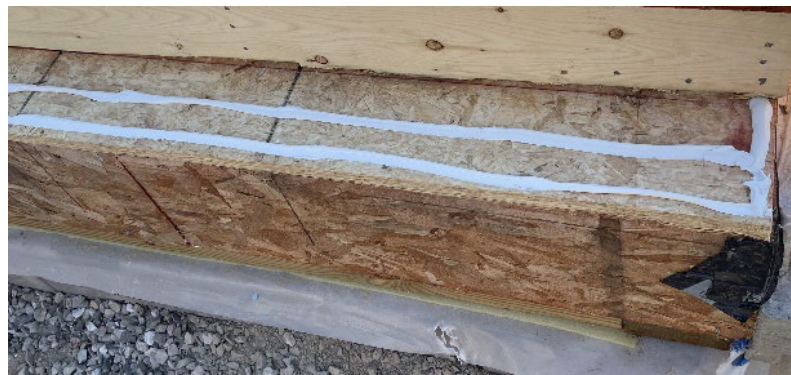
Figure 5-2. Air Sealing Caulk.
