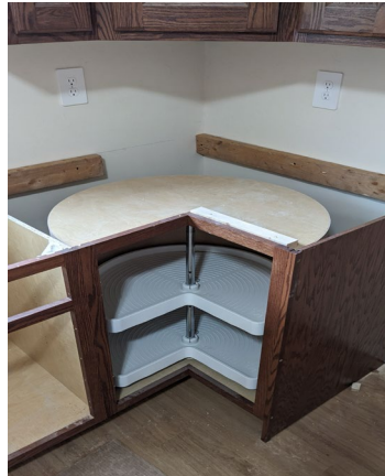
Figure 17-3. Showing Countertop 2x4 Corner Supports.
