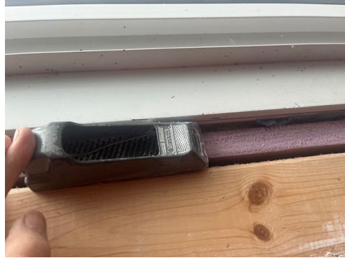
Figure 14-1. Trimming Foamboard Around Basement Window.
