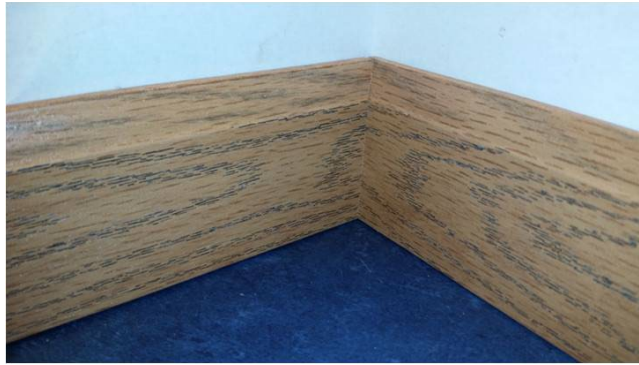
Figure 19-9. Finished Coped Joint.
