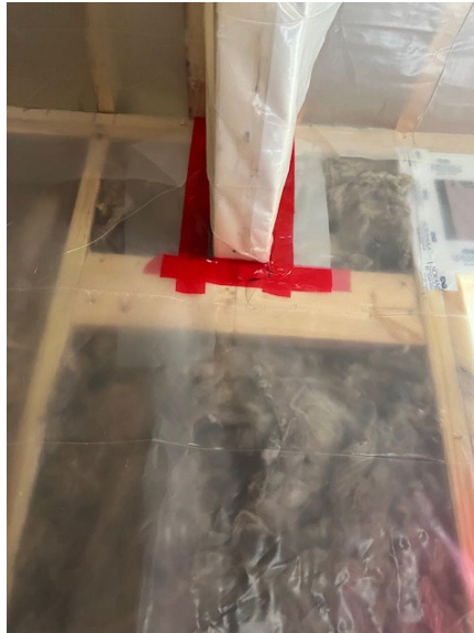
Figure 12-12. Air Sealing Around a Flush Closet Header.
