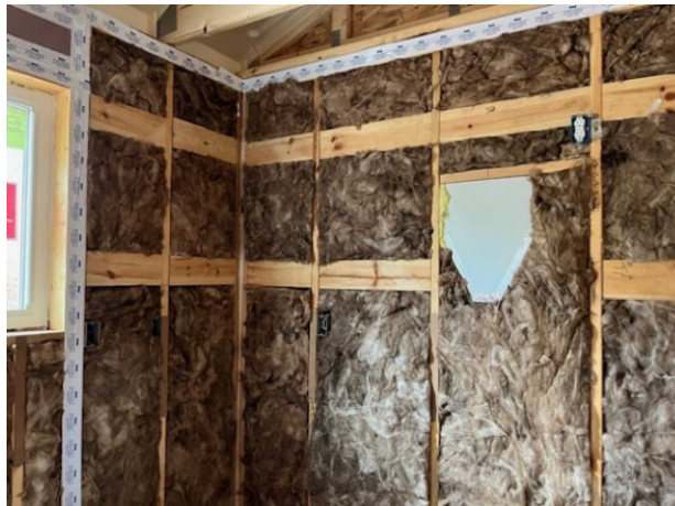
Figure 10-4. Kitchen Cabinet Blocking
