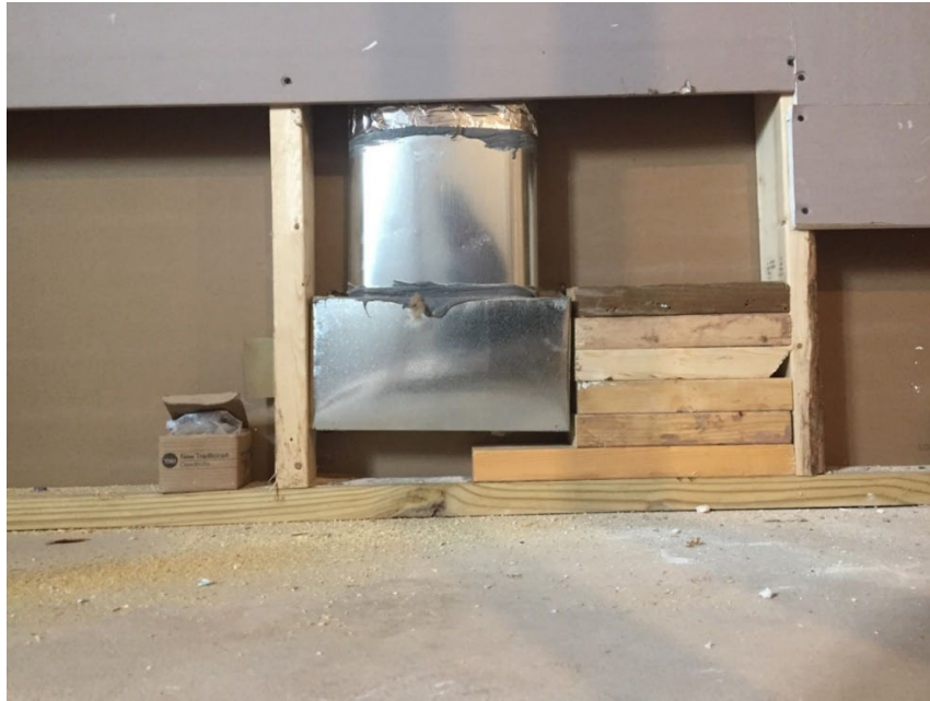
Figure 10-10. Cold Air Return Blocking.
