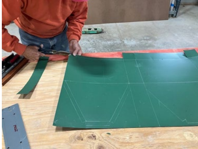
Figure C-5. Cutting Out Plenum Blank.
