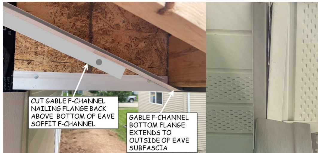
Figure 11-6. F-Channel at Gable Corner.
