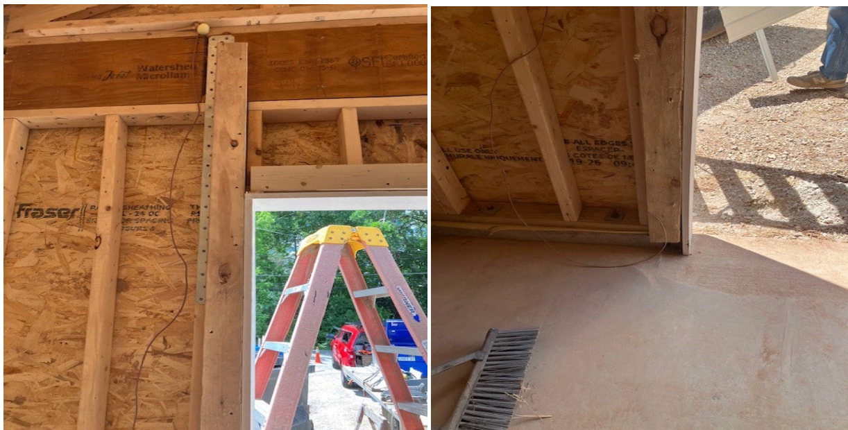
Figure 10-12. OHD Edge Blocking.
