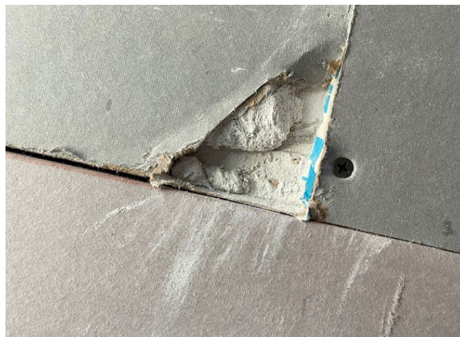
Figure 13-3. Broken Corner.
