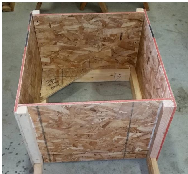
Figure 7-3. House Scuttle Box.
