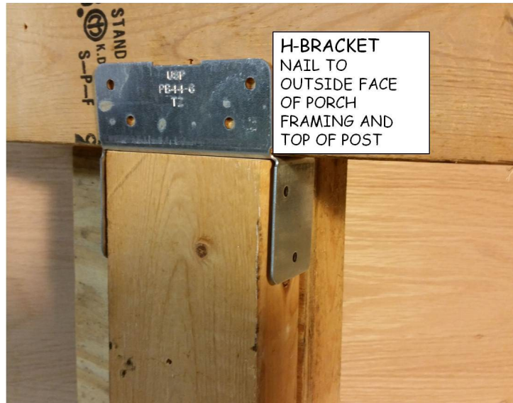
Figure 6-2. Porch Post H-Bracket.
