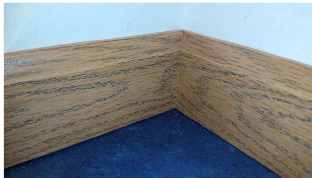
Figure 19-5. Finished Coped Joint.
