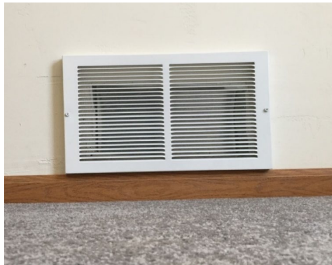
Figure 19-8. Positioning Cold Air Return Vent Covers.
