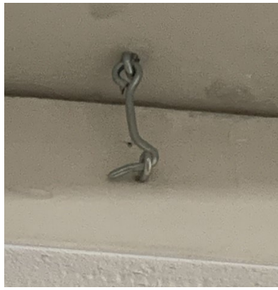
Figure 19-9. Garage Scuttle Cover Hook and Eye Assembly.
