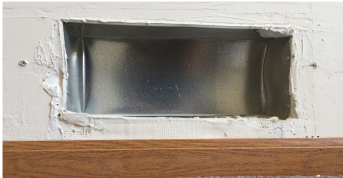
Figure 19-7. Sealing Plaster Gaps Around Cold Air Returns
