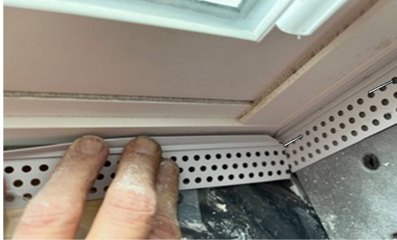
Figure 14-5. 45° Clipped Corners and Inside Row Hole Stapling.
