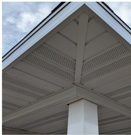
Figure 11-16. Porch Soffit Corner.
