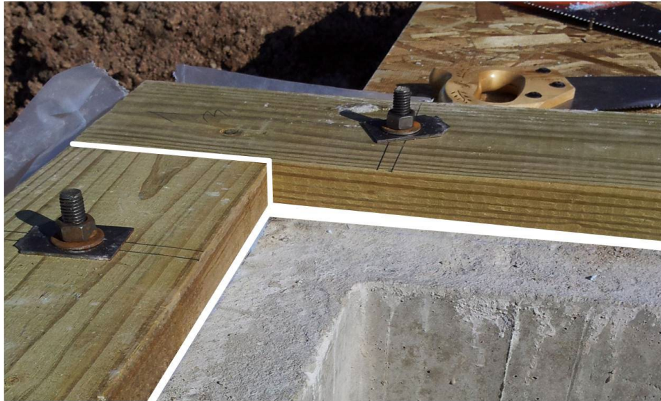
Figure 1-3. Sill Plate Installation.
