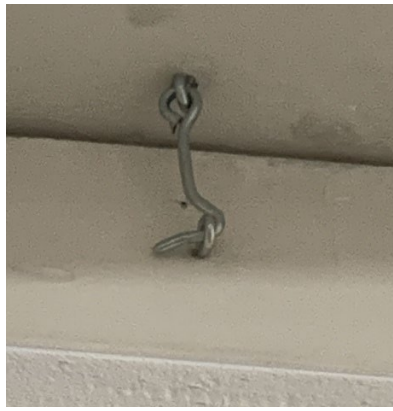
Figure 19-9. Garage Scuttle Cover Hook and Eye Assembly.
