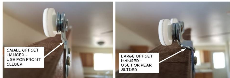
Figure 18-1. Sliding Door Hangers.
