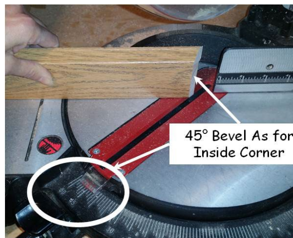
Figure 19-1. Base Trim Bevel Cut.
