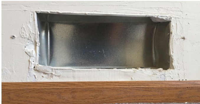
Figure 19-7. Sealing Plaster Gaps Around Cold Air Returns
