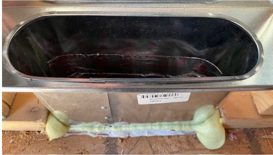
Figure 12-5. Sealing Cold Air Return Joints
