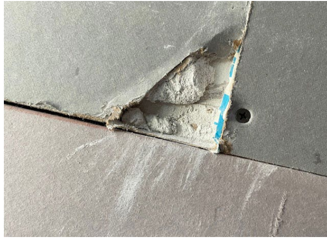
Figure 13-2. Broken Corner.
