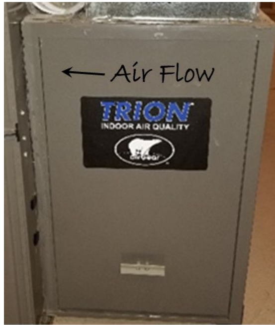
Figure 21-1. Furnace Air Flow Direction.
