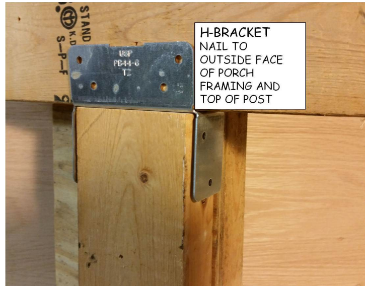
Figure 6-2. Porch Post H-Bracket.
