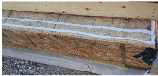
Figure 5-3. Air Sealing Caulk.
