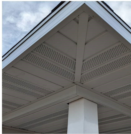
Figure 11-16. Porch Soffit Corner.
