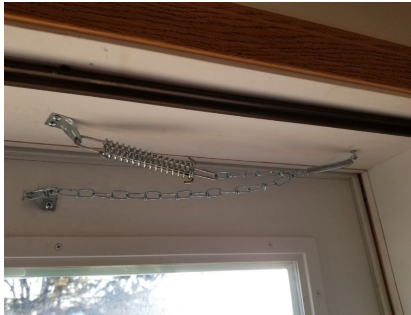
Figure 20-1. Storm Door Wind Chain.
