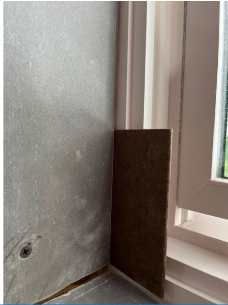
Figure 14-4. Shimming for Edging Strip Gap.
