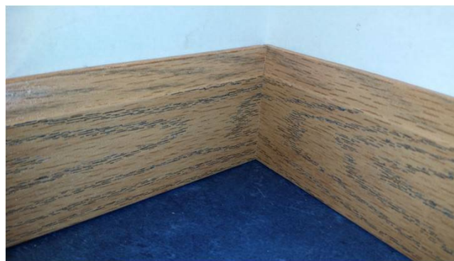
Figure 19-5. Finished Coped Joint.
