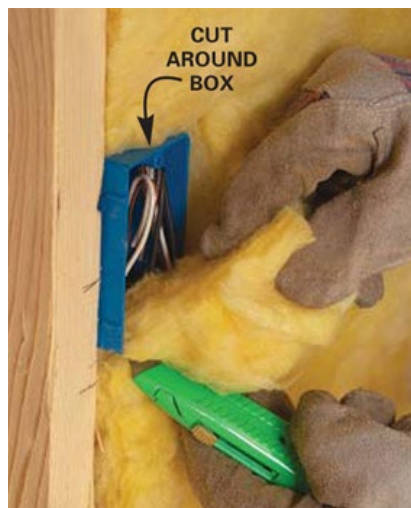
Figure 12-7. Insulating Around Electrical Box.
