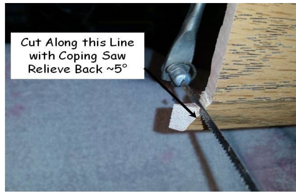
Figure 19-4. Coping Saw Cut.
