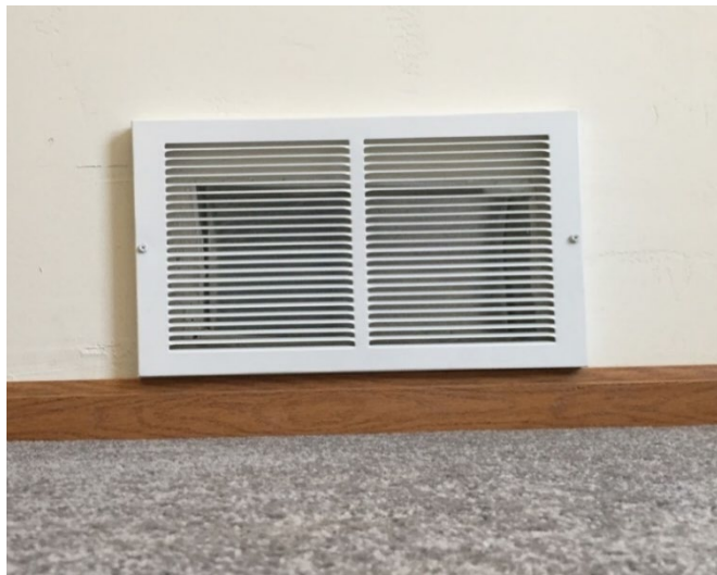
Figure 19-8. Positioning Cold Air Return Vent Covers.
