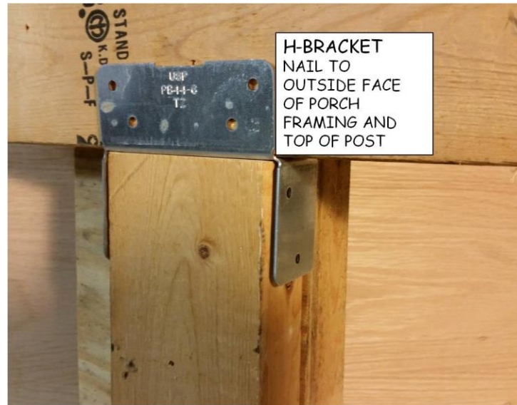
Figure 6-2. Porch Post H-Bracket.
