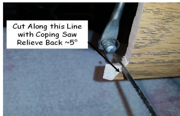
Figure 19-4. Coping Saw Cut.
