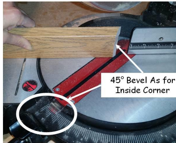
Figure 19-1. Base Trim Bevel Cut.
