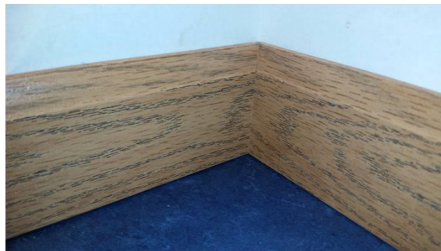
Figure 19-5. Finished Coped Joint.
