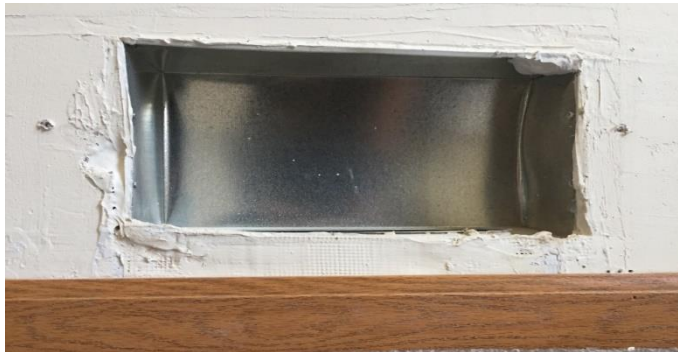
Figure 19-7. Sealing Plaster Gaps Around Cold Air Returns
