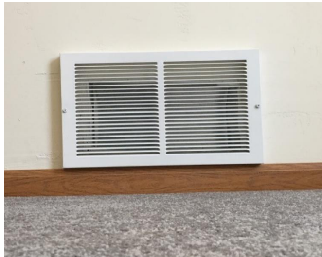
Figure 19-8. Positioning Cold Air Return Vent Covers.
